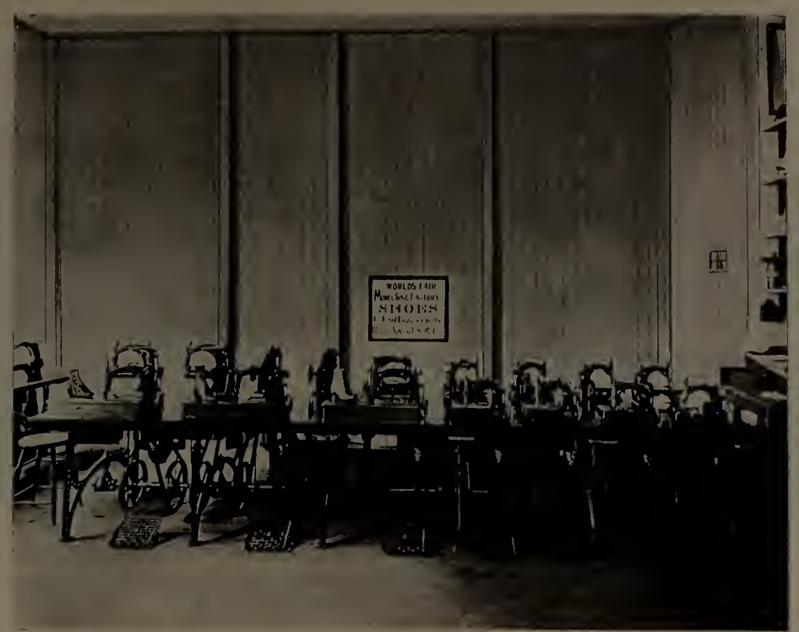
SALESROOMS OF THE UNION SPECIAL SEWING MACHINE COMPANY, 17 South Street.
